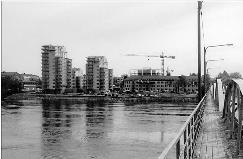
Fig. 4: New buildings on the brewery real estate in Umeå (Photo: Krister Olsson).
