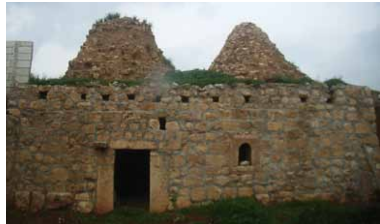
Fig. 18: Mud-stone technique in Aleppo (Saint Simon).
