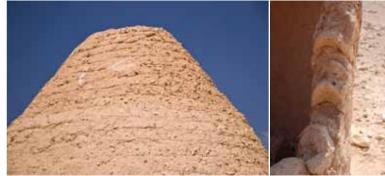
Fig. 17a: Cob technique in Idlib (Giobas). Fig. 17b: Detail of cob technique in Idlib (Giobas).
