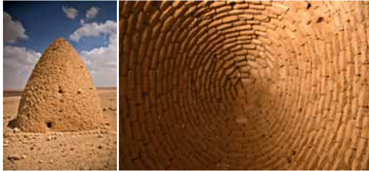
Fig. 16a: Earthen brick technique (adobe) in Hama region (Salamiyah). Fig. 16b: Earthen brick technique (adobe) in Hama region (Salamiyah).
