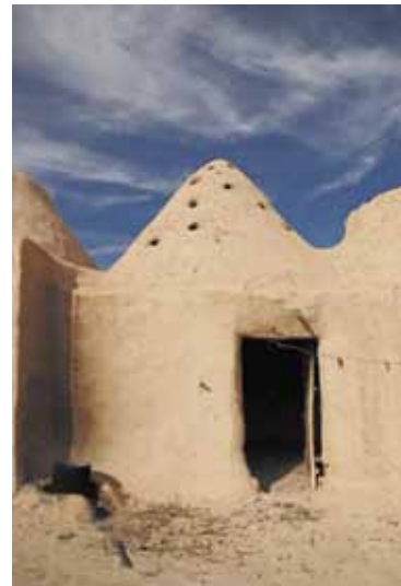
Fig. 23: Triangular Domes in Euphrates region. Fig. 24: Sultan domes in Hama region.
