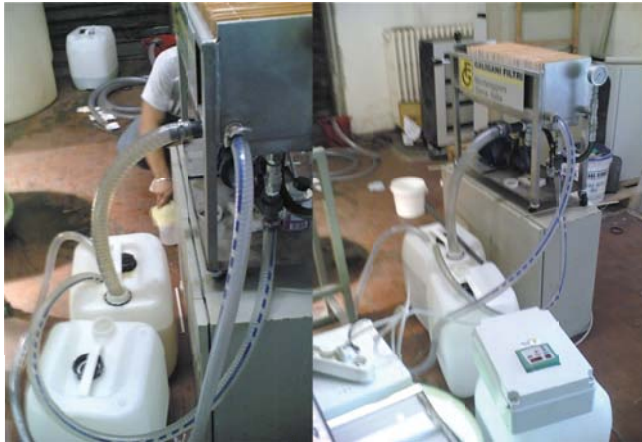
Figure 60: Details of the filter press. Left: detail of the inlet tube, at the left, recognizable by the yellow colour of the Cr(VI) solution at its interior, and the outlet tube of the filter press, white, through which the solution flows after reaction with biomass. Right: panoramic view of the filter press. In foreground the control unit and in the background inlet and outlet tubes of the filter press.
