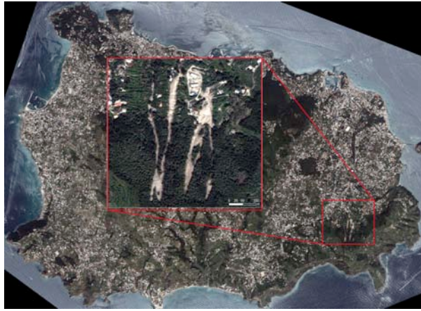
Figure 9.7: Localization of the Northern side of Monte Vezzi, where four debris flow occurred between 06:00 and 8:00 of 30th April 2006.
