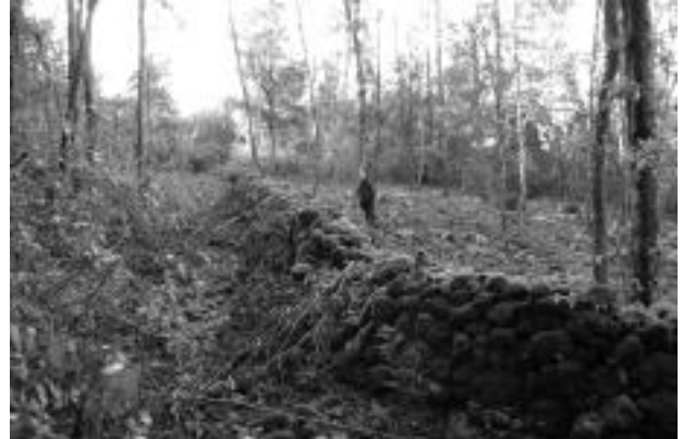
Fig. 10 - Section of self-standing dry stone wall made visible by forest harvesting activities.
