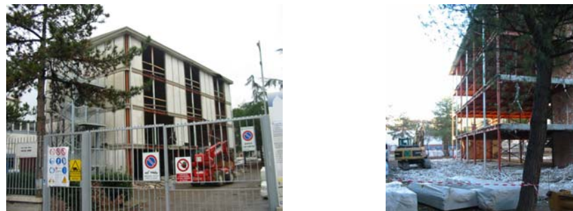
Figure 4. Views of the building during the demolition phases of the infills
