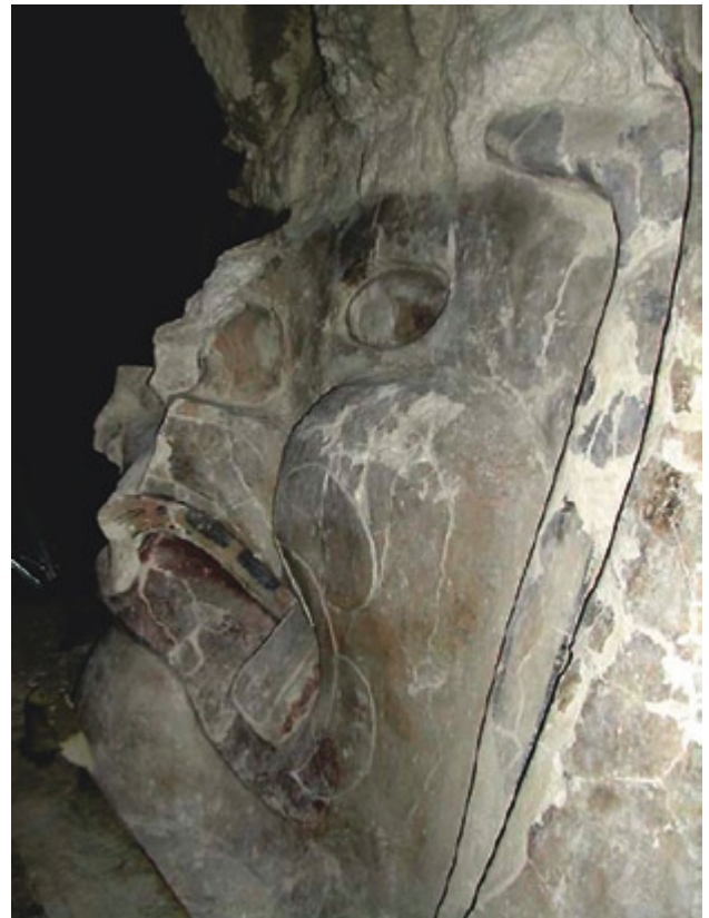
Fig. 3 Polychrome-modelled stucco mask in the sub-structure II c-1, in the inner part of structure II. The image was taken after re-adhesion of several detached fragments using autogenously air-setting mortar.
