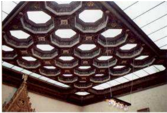
Internal view of atrium: the original roof “a cassettini”
