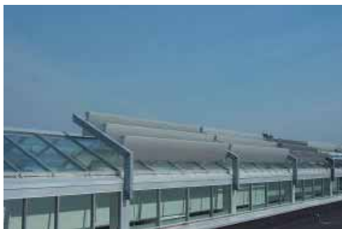
Figure 5 Shading devices at Aabenraa Hospital.
