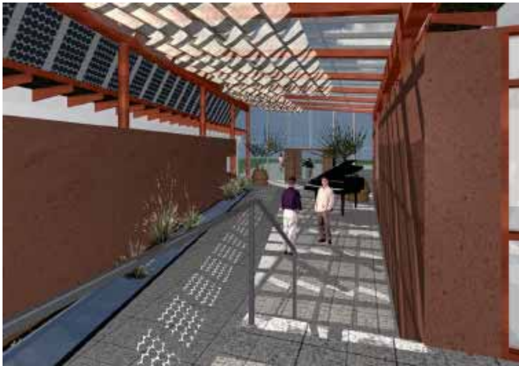
Figure 6 Fachkrankenhaus Nordfriesland Hospital The large ceiling surface has a shallow north facing slope; here a white curtain is used to reduce solar radiation. On the south facing steeply sloping roof section, polycrystalline PV modules are integrated into the glazing to act as solar shading while generating electricity.
