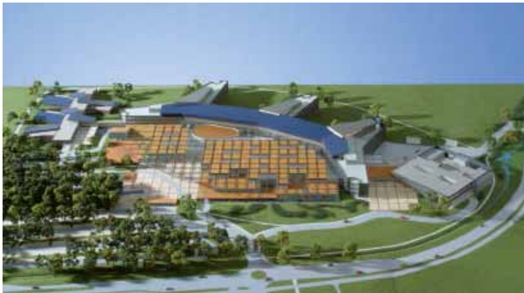
Figure 1 View of Deventer Hospital
