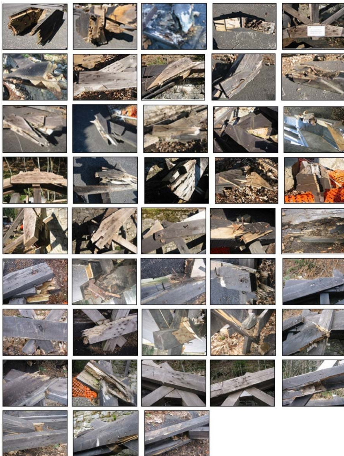
Image 6. The 43 joints found in the rubble
