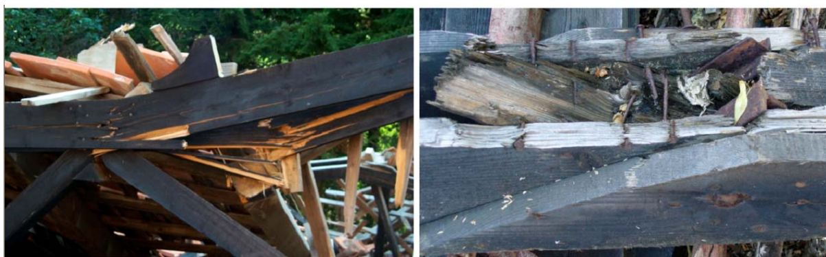
Images 4–5. Joint "E" or "C" (left) and heel joint "A" or "G" (right), respectively ductile and brittle failures. Brown-rot decay was in the heart of heel connection ("A" or "G").
