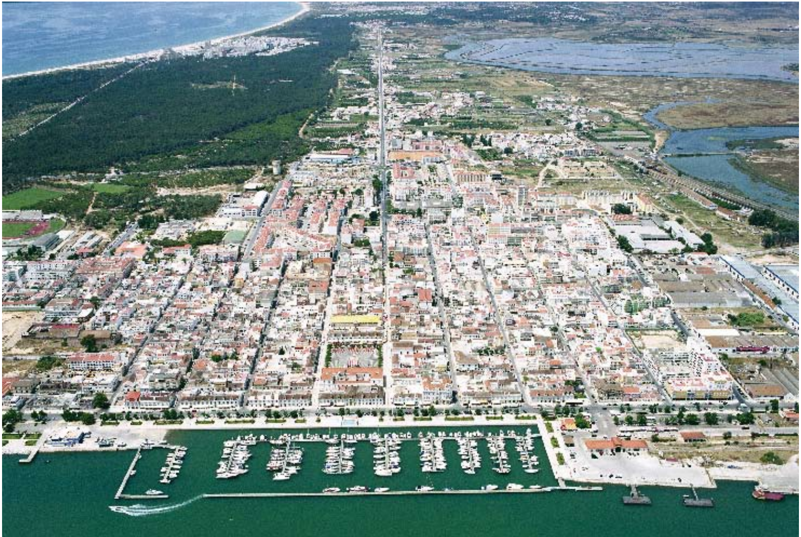
10. Aerial View of Vila Real
