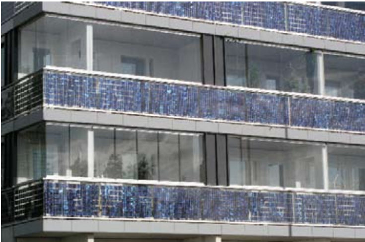
3. Ecological experiments relating to the utilisation of solar energy and new ventilating systems
