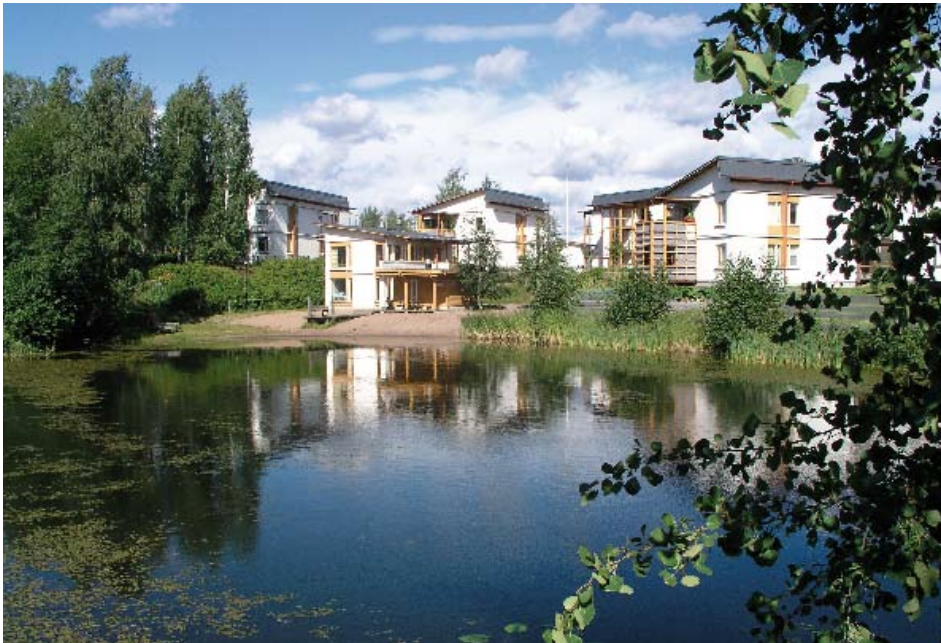
5. Experimental area for timber construction apartment buildings
