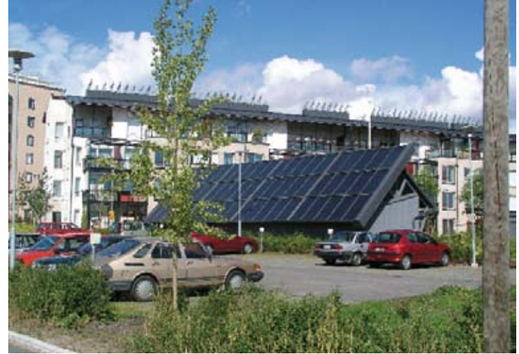
2. Finland's first apartment building using solar electricity. Panels are located on balconies
