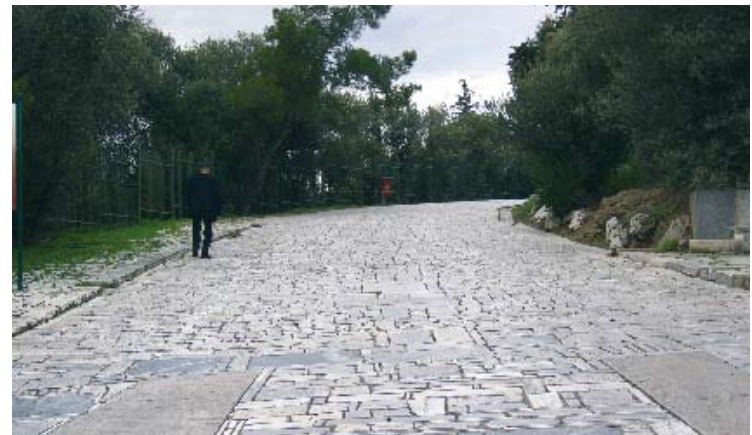
2. Details of the Pichionis project
