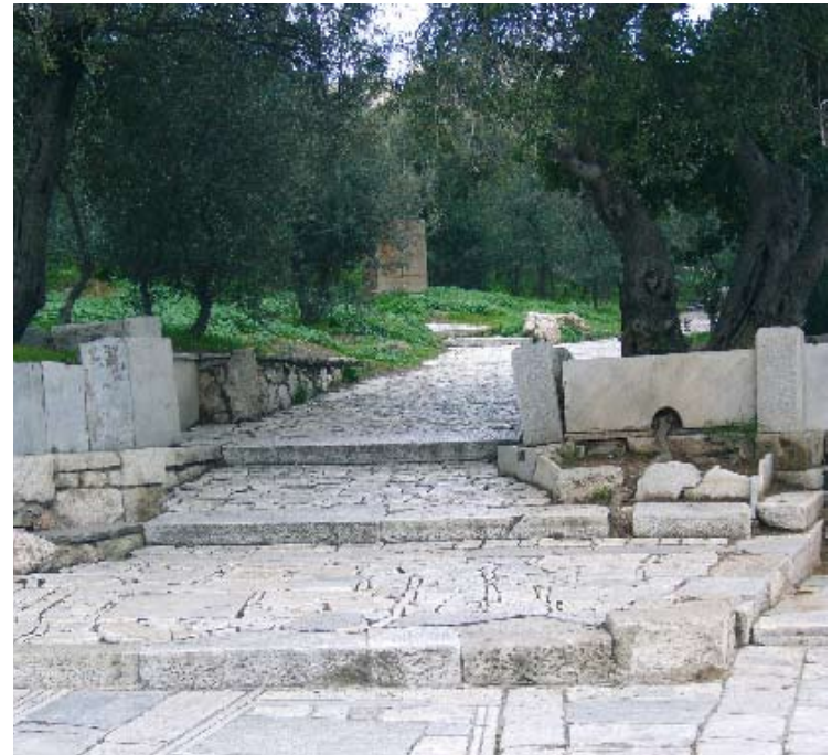
5. Details of Pichioni's works
