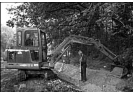
Figure 2. Restoration of loam layer to keep the 'spreng' (manmade water channel) waterproof
