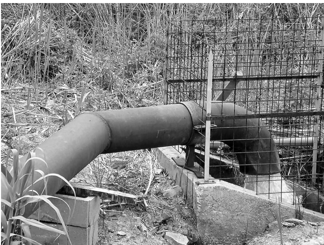
Figure 15. Water pumping system at the Gavorrano underground mine (at present, about 80 L/s)
