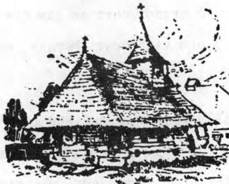
Wooden Church in Moisei, Transylvania
