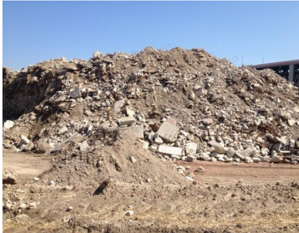
Figure 14 - Waste material stockpiled at Carter Road Site
