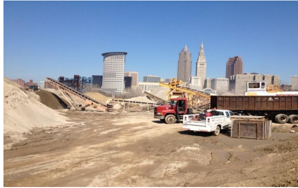
Figure 13 - Independence's Carter Road mobile crushing plant
