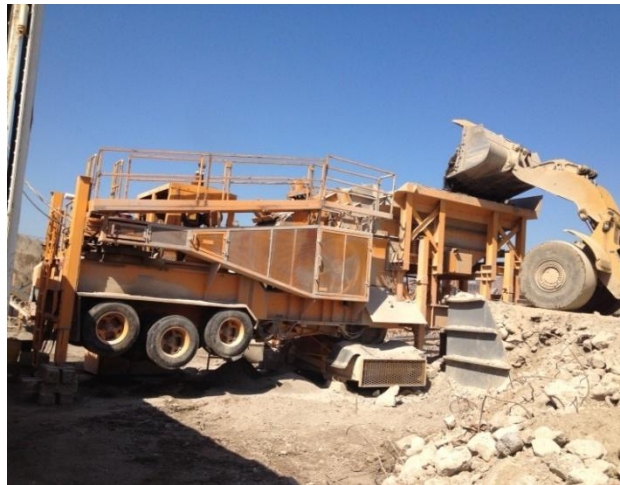
Figure 16 – Demolition material being loaded into horizontal impact crusher
