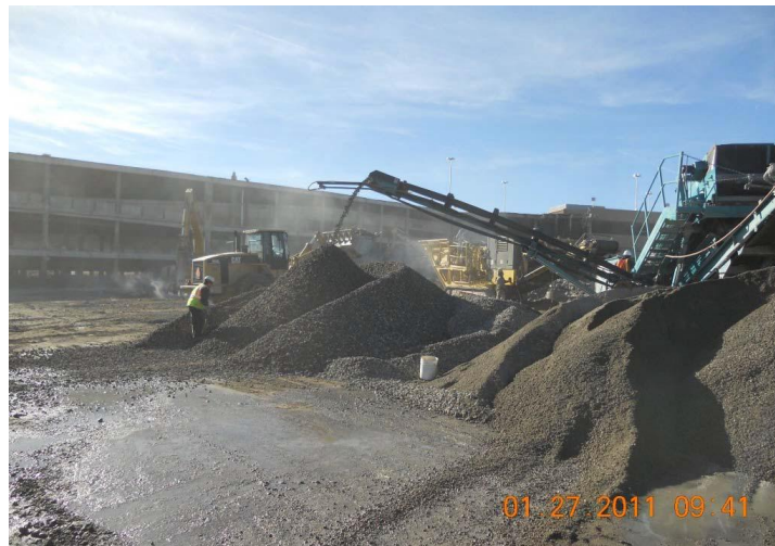
Figure 23 - Recycling of Construction Debris at Stapleton Airport
