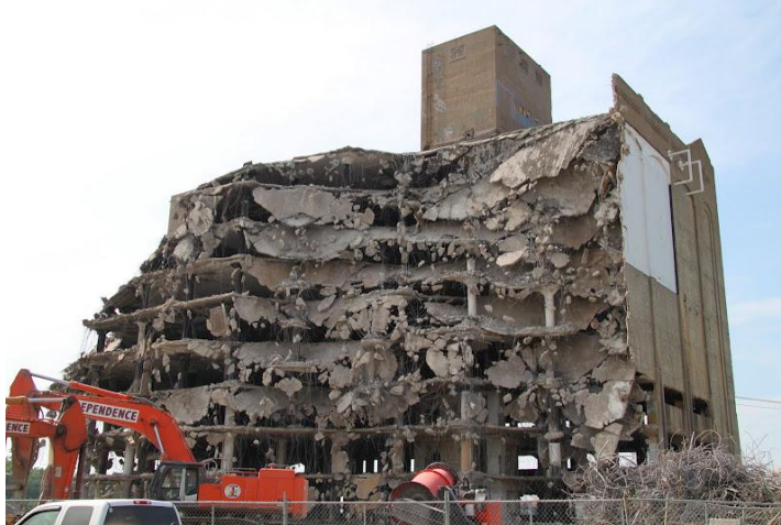
Figure 12 - Demolition of the Cleveland Cold Storage Building
