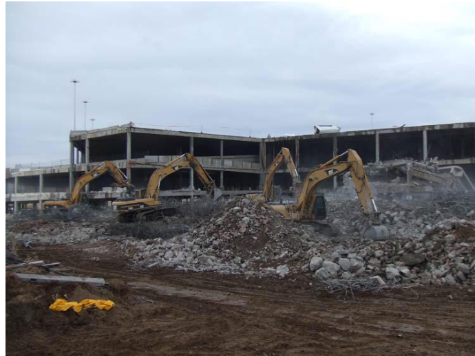
Figure 22 - Demolition of the Stapleton Airport Parking Garage
