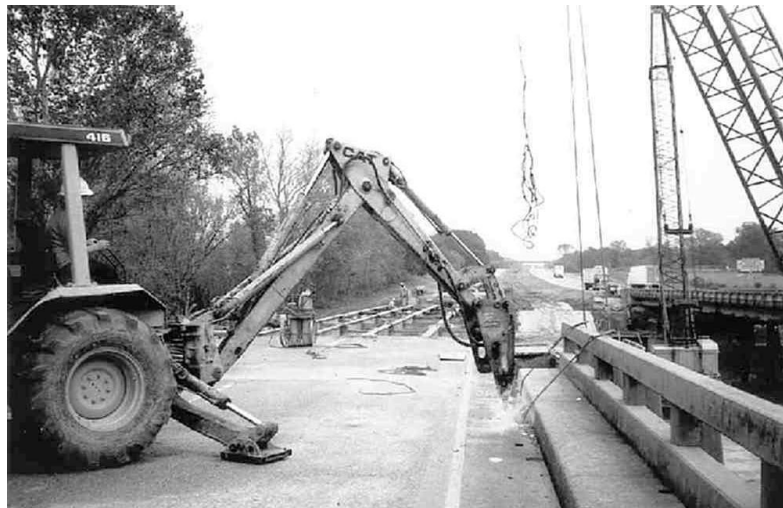
Figure 2 - Vehicle mounted impact breaker (ACI 555, 2011)
