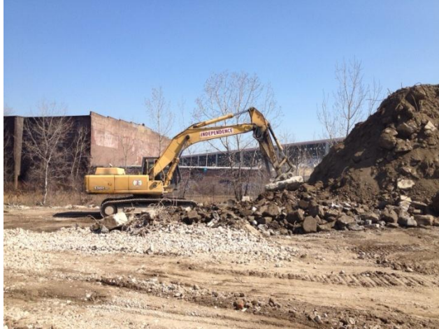
Figure 15 - Processor separating demolition material
