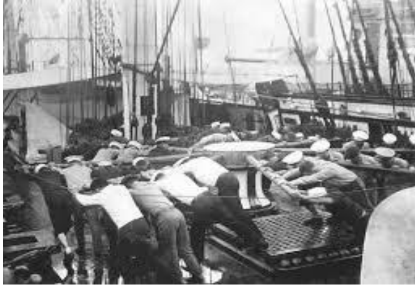
Figure 5. The capstan on the USS Constitution . Reprinted from Brown & Harfiled's Capstan by Friends of the Capstan, Inc. (n.d.) Retrieved June 29, 2015 from www.cerberus.com.au/capstan.html
