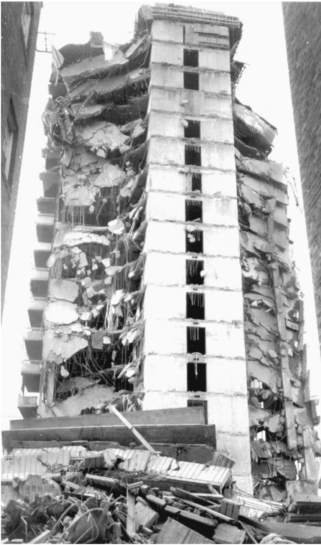
Fig. 2. Building collapse; four men missing and three injured when apartment under construction collapsed in Brighton [from Boston Globe , January 26, 1971; republished with permission]
