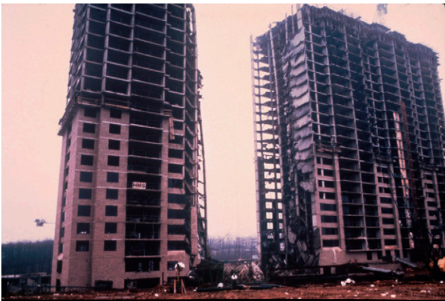
Fig. 2. The collapsed structure (courtesy of NIST)
