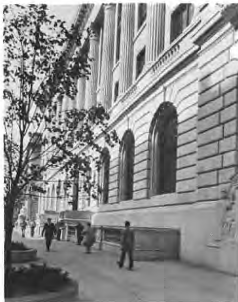
Main building of the Cleveland Public Library at 325 Superior Avenue, scene of pioneering adaptation of computers to library cataloguing.
