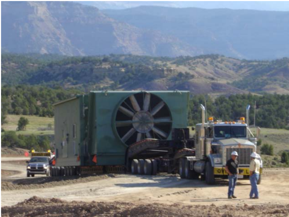
Figure 8. Compressor being installed (Courtesy of M3 Midstream, LLC)
