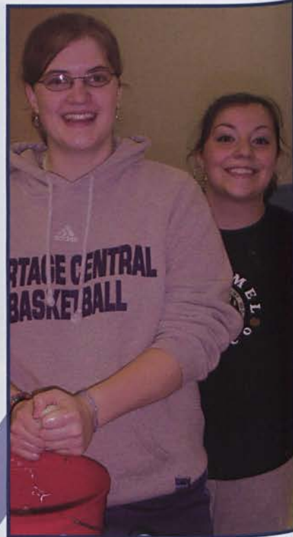
Cori Ginter and Jamie Anderson help paint the second floor of ICI in Chicago, which was under construction and slated to become a whole floor dedicated to afterschool Bible lessons during the week and on Sundays.
