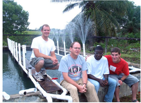
The fountain spray cooling system designed and built by seniors for their capstone design project . Ten spray heads on a 30' line were sufficient to dump more than 60 kW of heat. Each head was machined with 78 0.043" diameter holes at four different angles to get an oval spray pattern. (right) The two graduates and their Liberian helper Patrick who built the cooling system.
