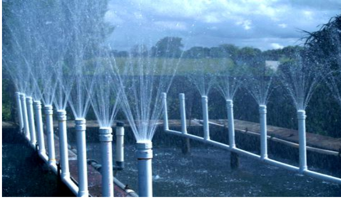
The fountain spray cooling system designed and built by seniors for their capstone design project . Ten spray heads on a 30' line were sufficient to dump more than 60 kW of heat. Each head was machined with 78 0.043" diameter holes at four different angles to get an oval spray pattern. (right) The two graduates and their Liberian helper Patrick who built the cooling system.
