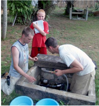
Students inspecting of one of many distribution boxes on campus. At these stations water pressure and flow rate measurements were taken and recorded. Occasionally budding engineers volunteered to help the students.
