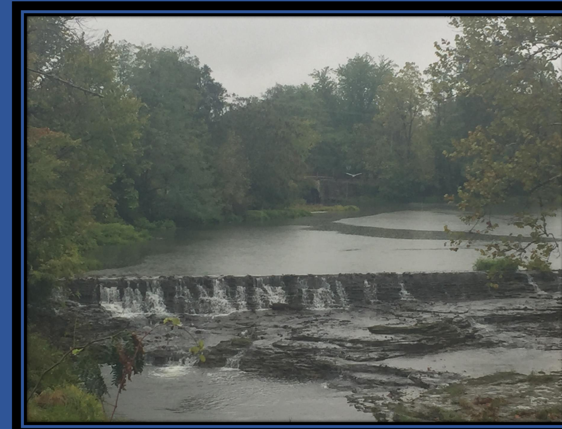
The view from in front of the overhead dam.
