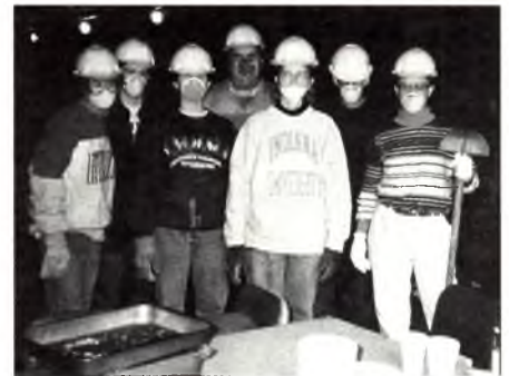
Indiana University Nazarenes don masks as they assist in a spring break demolition project in Boston, Mass.
