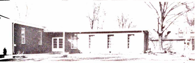
2 Benson Memorial Church of the Nazarene, Nashville, Tennessee, recently dedicated its new church building, consisting of a sanctuary on the left which will seat 150 persons, and an educational unit on the right with six classrooms, church office, and rest rooms. Wallace Churcher, Nazarene layman, was the contractor for the structure, with the total property valued at $35,000. Dr. C. E. Shumake, district superintendent, and Dr. W. T. Purkiser, Herald editor, participated in the service. Rev. William Strickland is the pastor.
