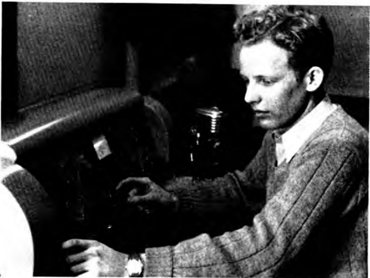
IN THE RADIO CONTROL ROOM
