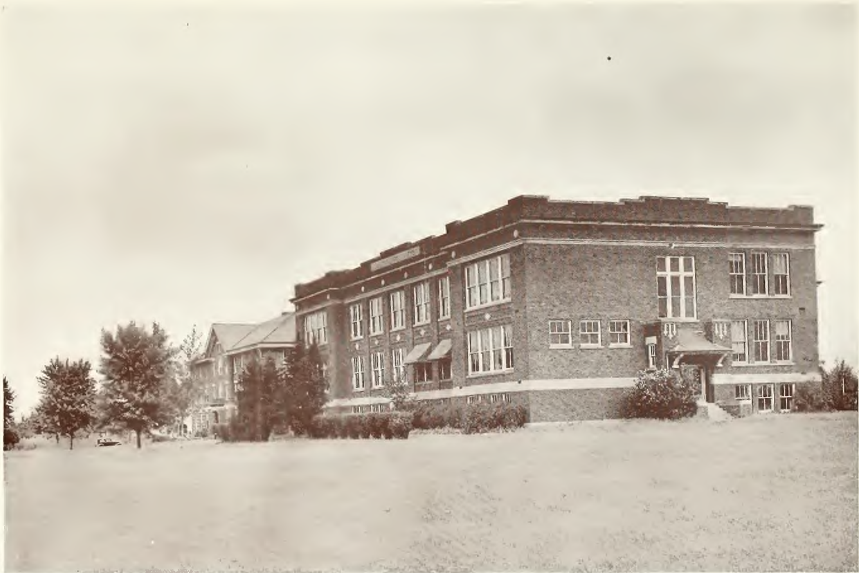
ADMINISTRATION BUILDING (South View)
