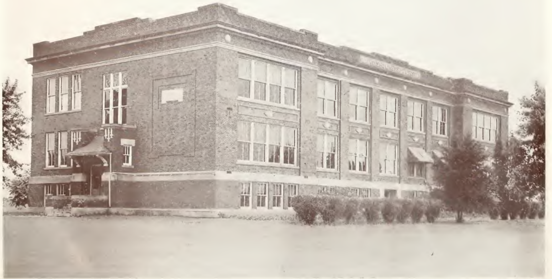
ADMINISTRATION BUILDING (North View)
