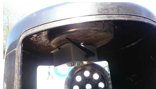
Figure 8. Sensor nodes are attached to the bins using simple mechanical fasteners.
