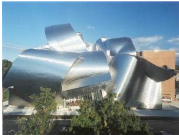
Figure 1: Peter B. Lewis Building at Case Western Reserve University
