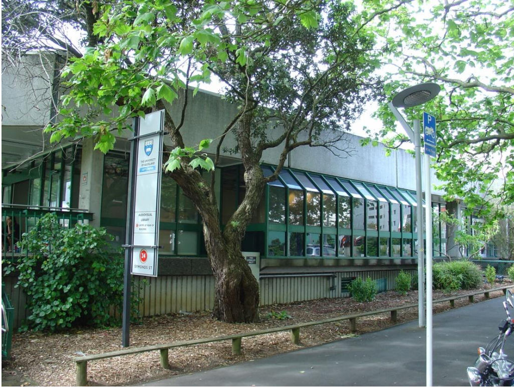
Fig 2: Computer Centre of the University of Auckland, Auckland, New Zealand (Photo: L. Janczewski)
