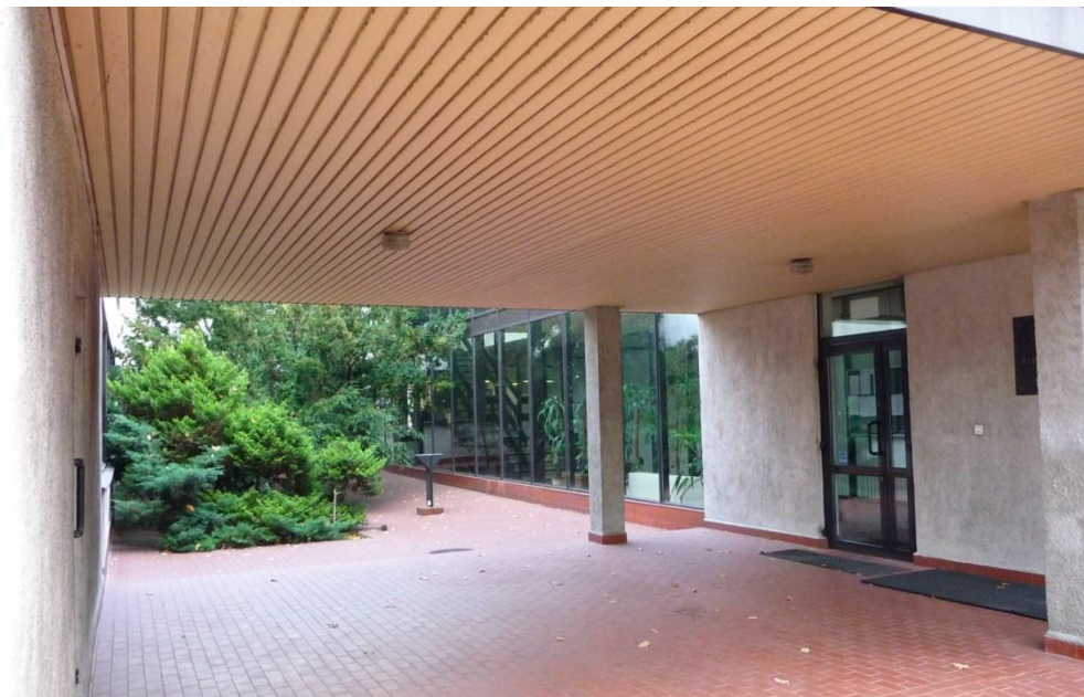
Fig 1: Former Computer Centre of ZETO-ZOWAR, Warsaw, Poland (Photo: L. Janczewski)
