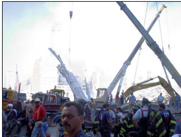
Figure 1. Heavy Equipment at Ground Zero
