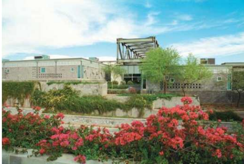
Figure 1: Solid Waste Transfer and Recycling Facility, Phoenix, Arizona, 1993
