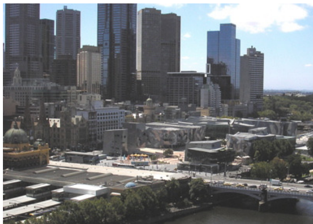
Figure 1: Federation Square, Melbourne, Australia
