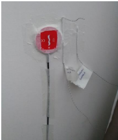
Fig. 12 – HFM and internal thermocouple fixed
