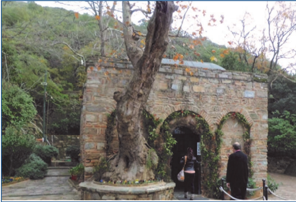
Photo 1: View of Entrance Gate of Mary Mary House (December 2012)
