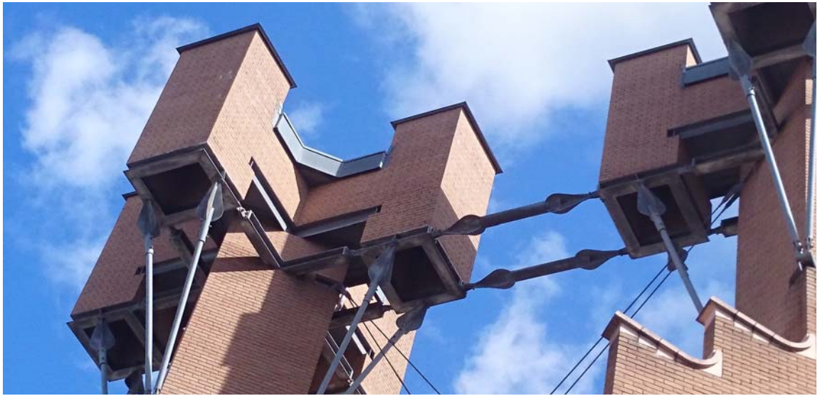
Figure 88: detail view of brick H-pots to studio theatre
