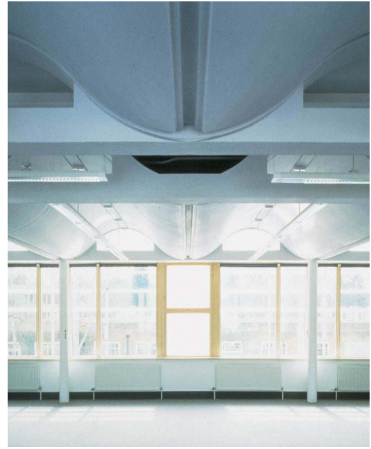
Figure 34: BRE office building interior; showing curved concrete soffit. (Feilden Clegg Architects)
