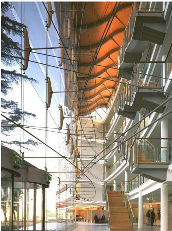
Figure 36: Fingal County Hall atrium. (Bucholz-McEvoy Architects 2000).
