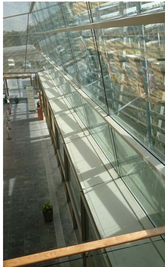
Figure 66: atrium showing actuator-driven louvre to base of glazing
