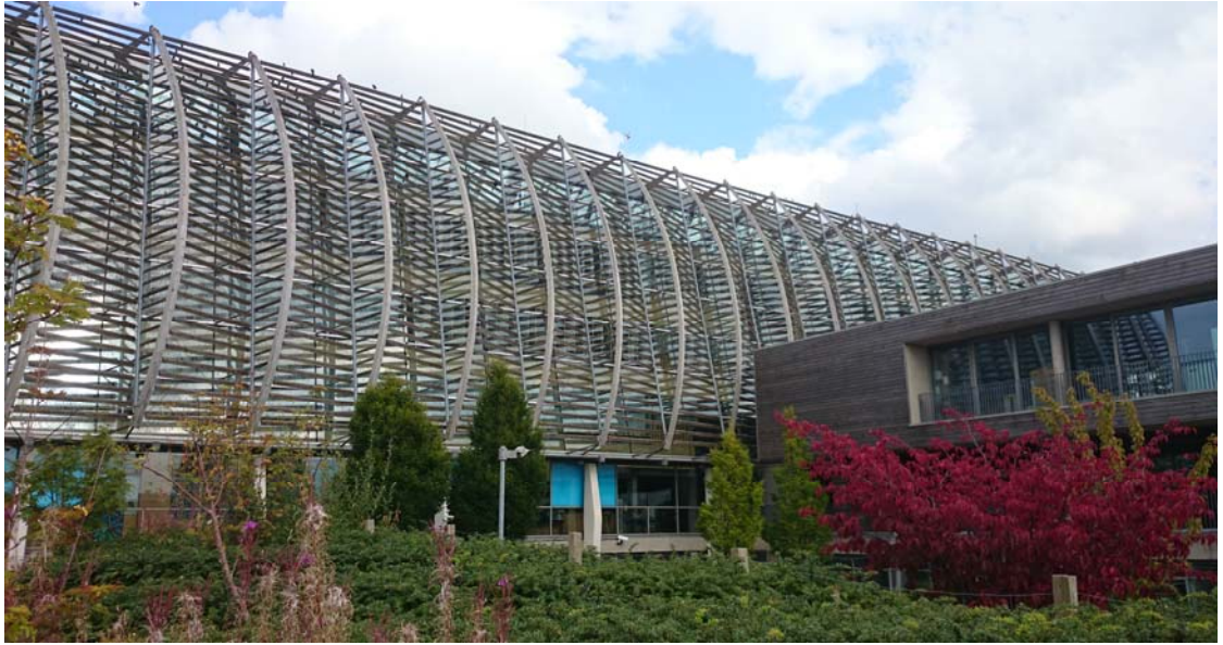
Figure 52: south west façade showing brise-soleil to the atrium
