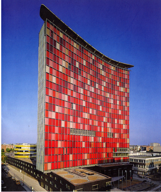
Figure 24: GSW Tower Berlin, double skin stack (Sauerbruch and Hutton)
