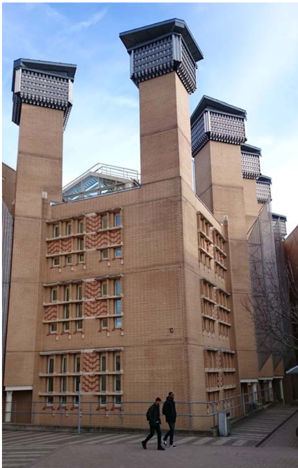
Figure 100: perimeter extract stacks
