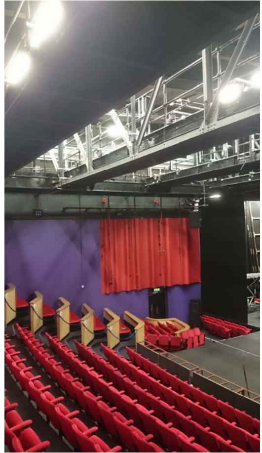
Figure 81: main auditorium space with lighting gantries and above them the ventilation stacks
