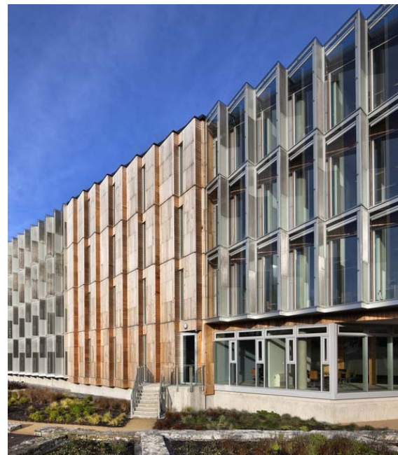
Figure 71: Westmeath County Council building – double skin façade to south elevation – (Bucholz-McEvoy Architects)
