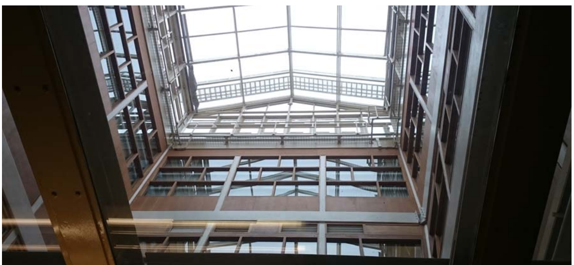
Figure 113: ground floor looking up into the central extract light well
