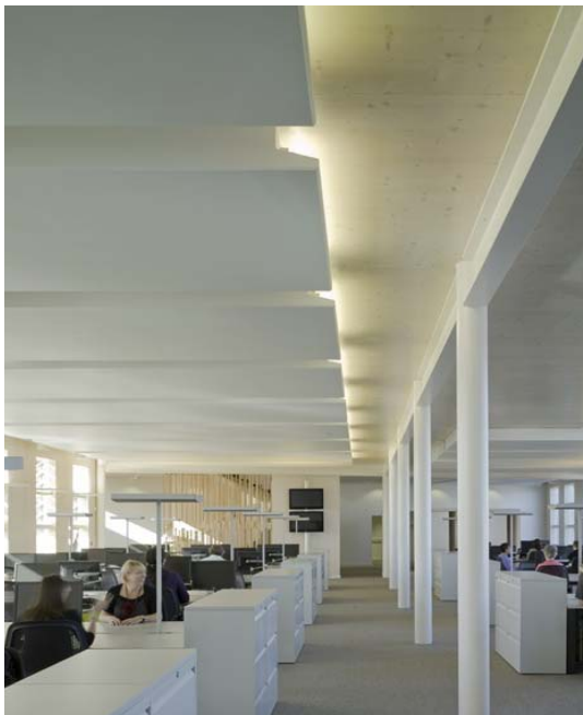
Figure 26: Thermal mass in ceiling deck at the Woodland Trust HQ. (FCB-Studios)
