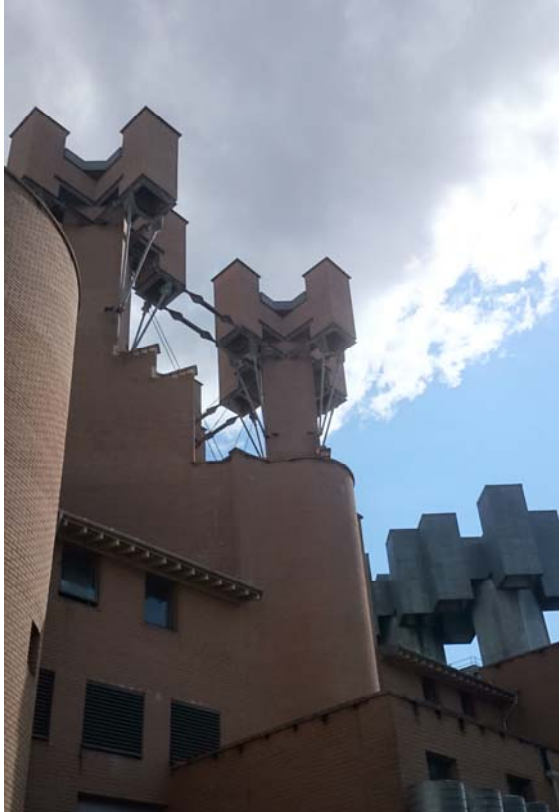
Figure 92: brick stacks to studio theatre
