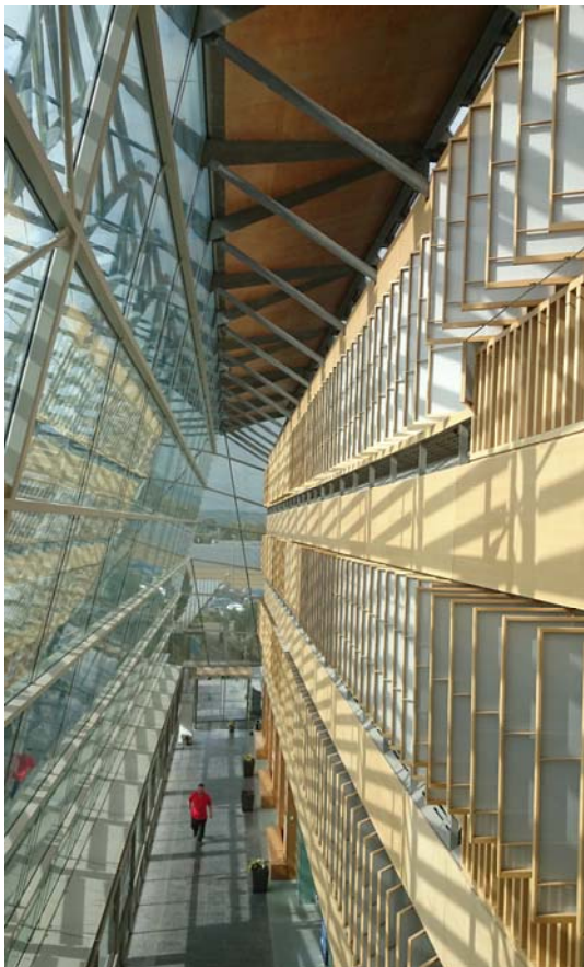
Figure 65: atrium showing light weight shutters to offices for light control
