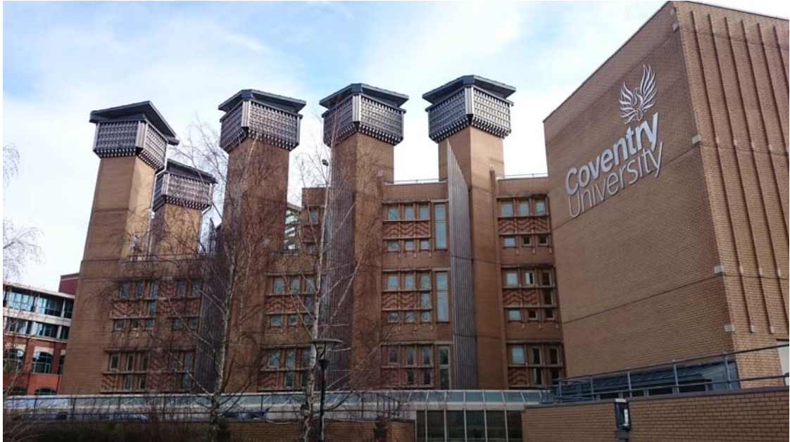
Figure 94: main entrance elevation to Lanchester Library
