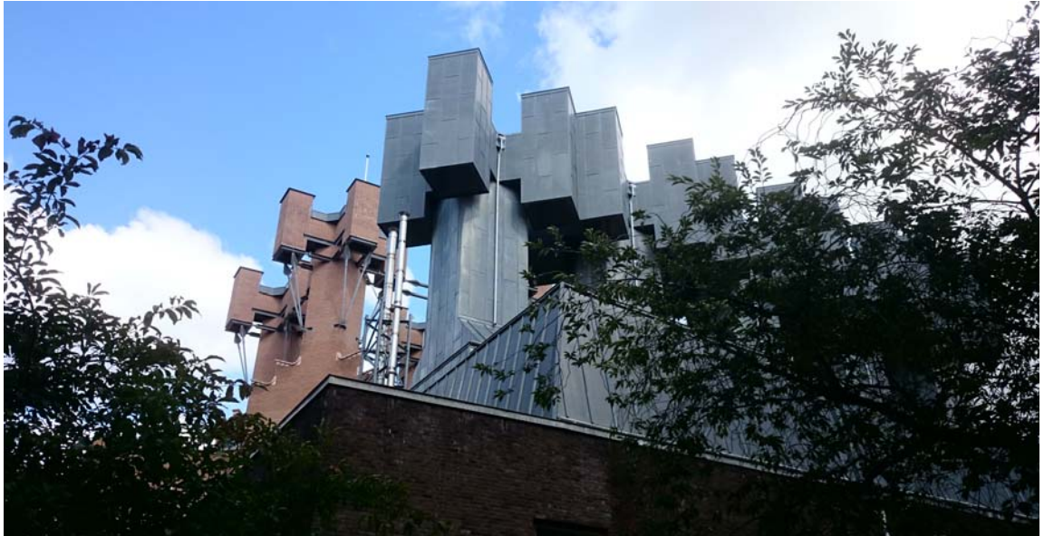
Figure 83: view from western courtyard with main theatre in foreground with zinc clad stacks and the brick stacks of the studio theatre beyond.
