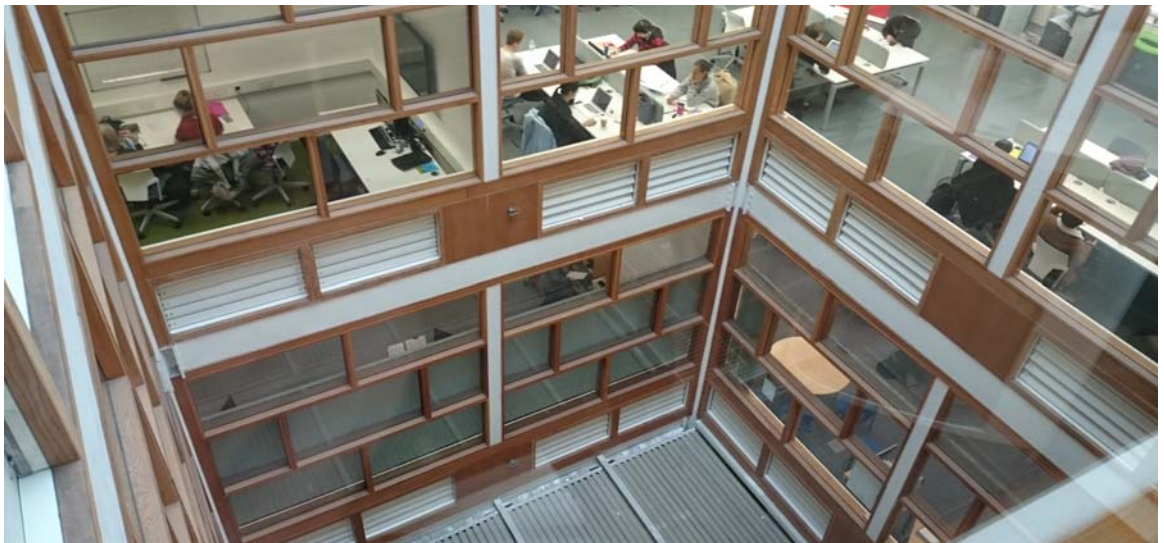
Figure 104: light well/ air ingress from above showing louvers into library spaces
