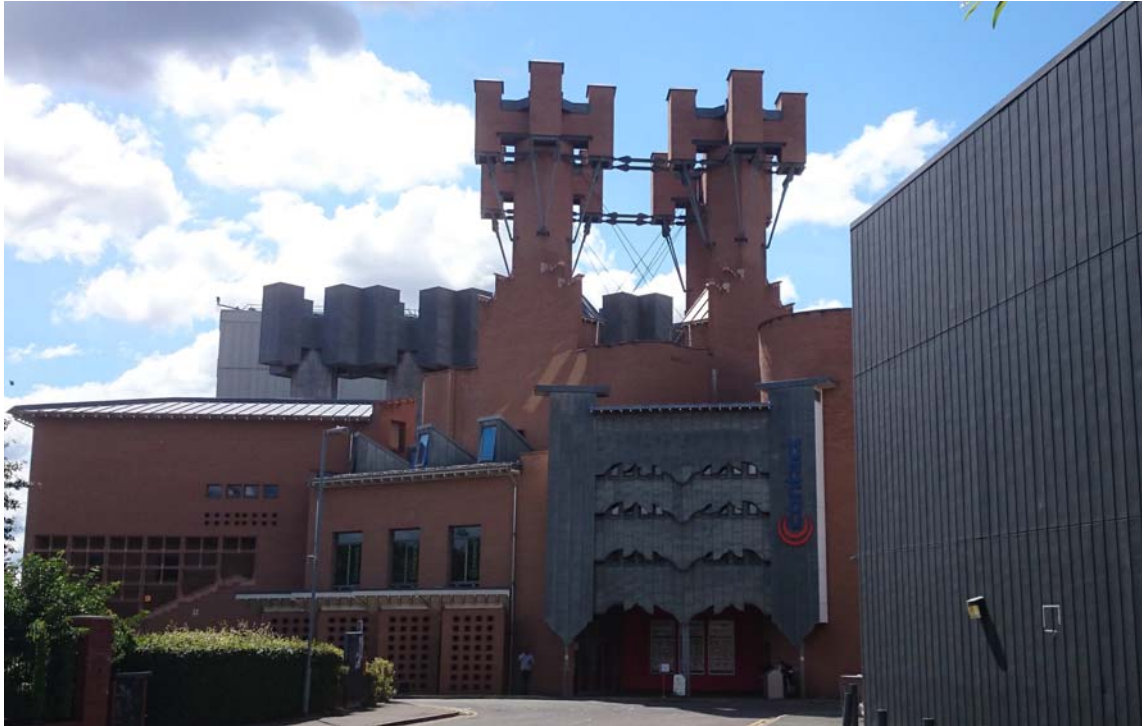
Figure 72: public entrance to the Contact Theatre, showing studio theatre stacks and behind the main theatre block with its dedicated zinc clad ventilation stacks.
