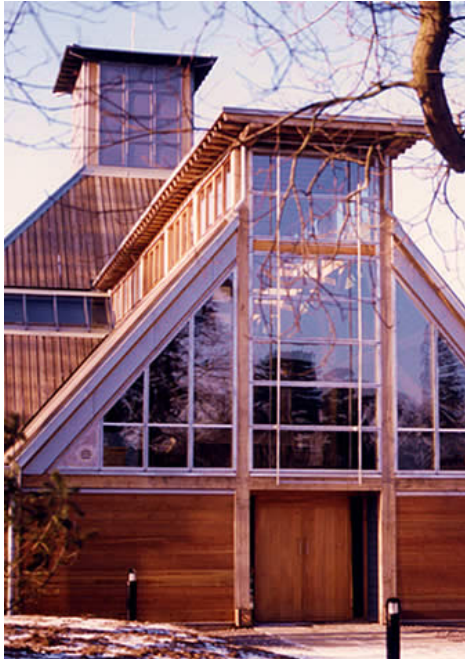
Figure 41: Bedales Theatre, UK; exterior view showing stack above auditorium. (Feilden Clegg Architects)
