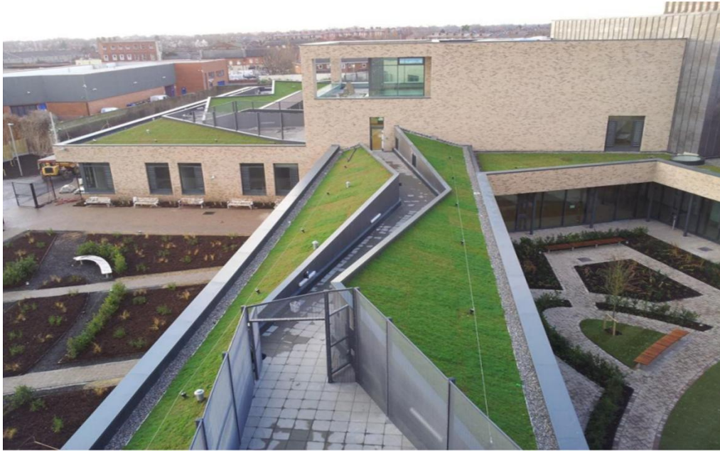
Figure 1: Example of green roofing at Grange Gorman
