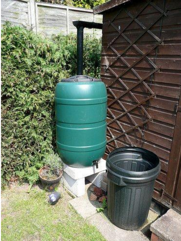
Figure 1.2: An example of rainwater harvesting in Ireland
