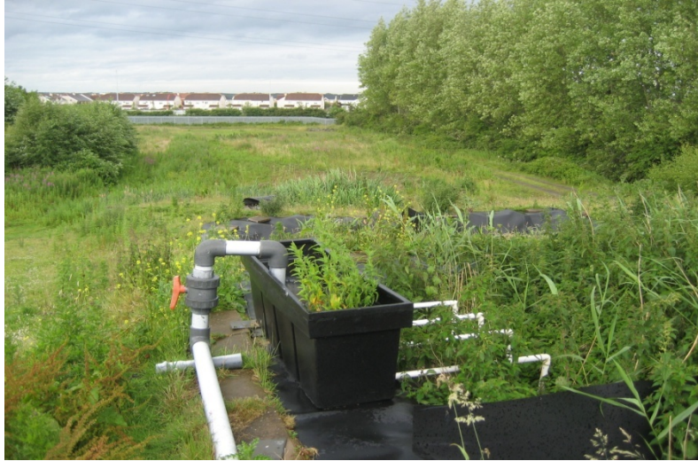
Figure 29 Primary vertical beds with weeds colonising the header tank and the bed
