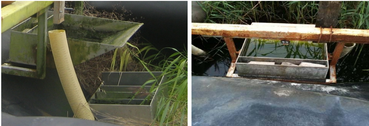
Figure 16 Tipping bucket system to SVF
