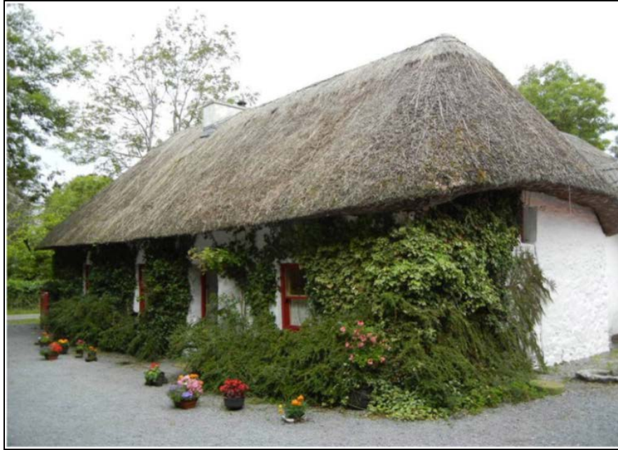
Figure 2: Cottage Rathbaun Farm Co. Galway
