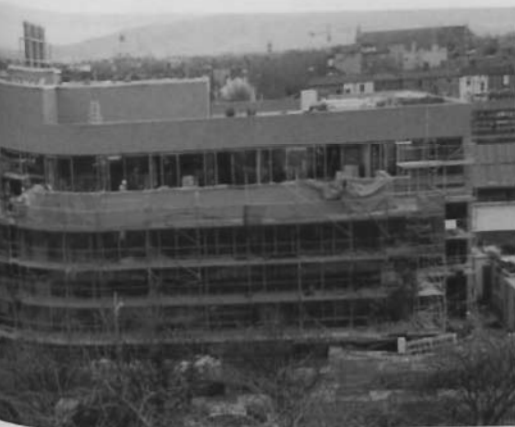
Completing from the roof downwards
