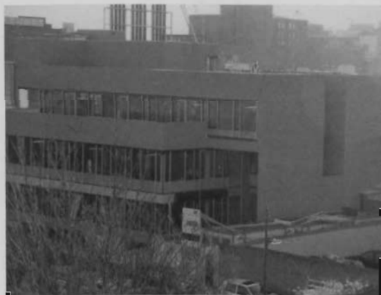
Close to finishing off in Spring 2004
