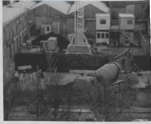
Foundation for the basement
