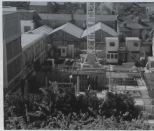
Building taking shape
