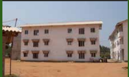
Below: Finished apartments in Panadura
