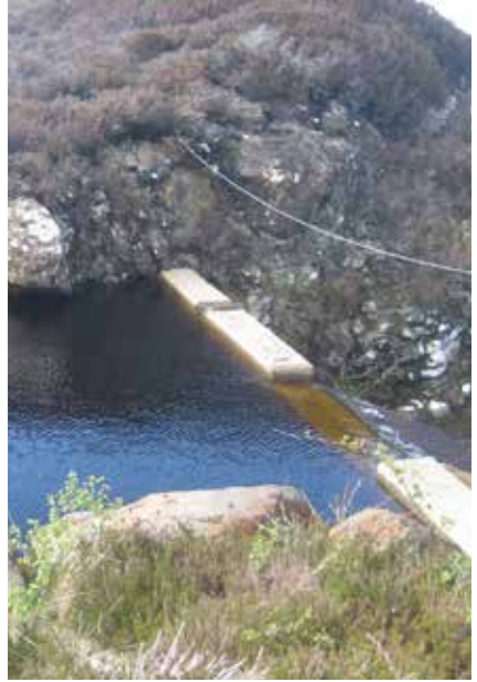
The new system involved damming the river high above the north western part of the island, and piping water down to a housed turbine. By using the moorland plateau a head for the water of 100 m was achieved.
