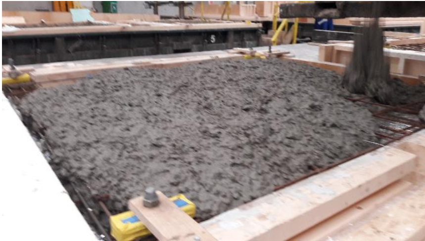
Figure 3. Prototype PCM panel under construction
