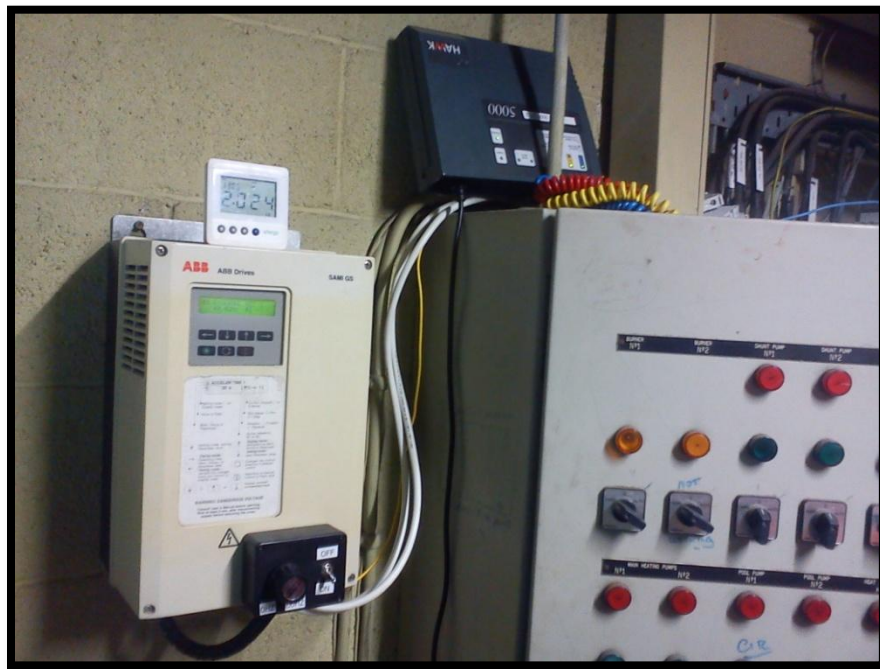
Figure 47: VSD installation
