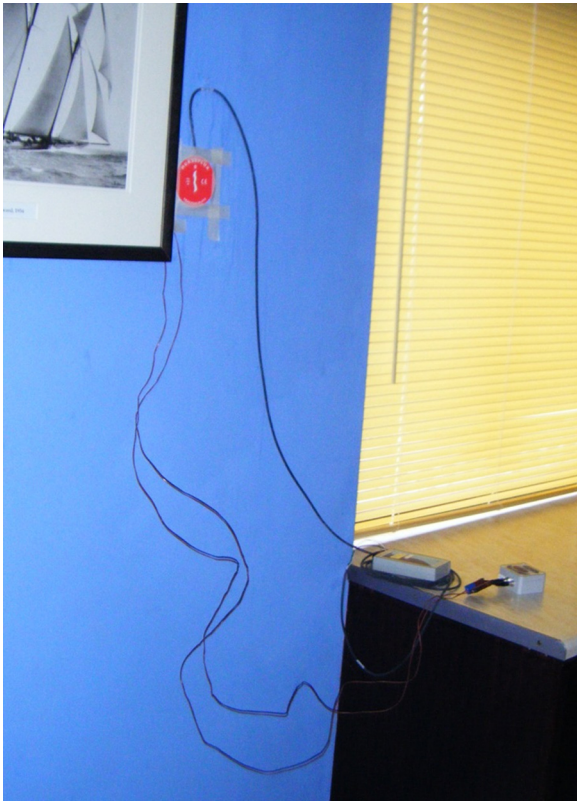
Fig. 2. Position of wall heat flux metre and internal surface temperature sensor.
