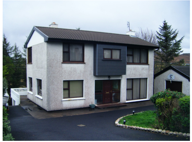
Fig. 1. View of case study building from the north-west.
