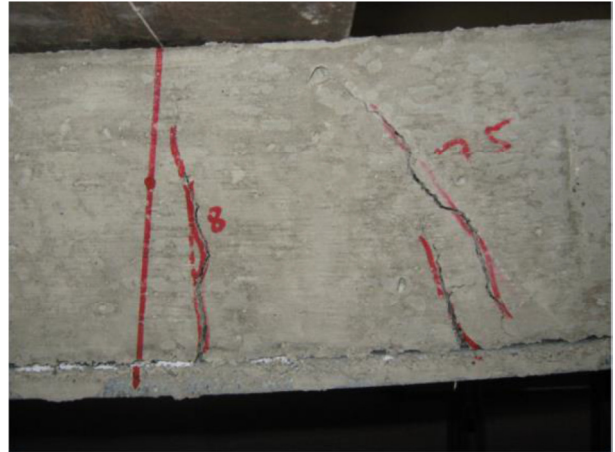
Diagonal Shear cracks – Right hand side
