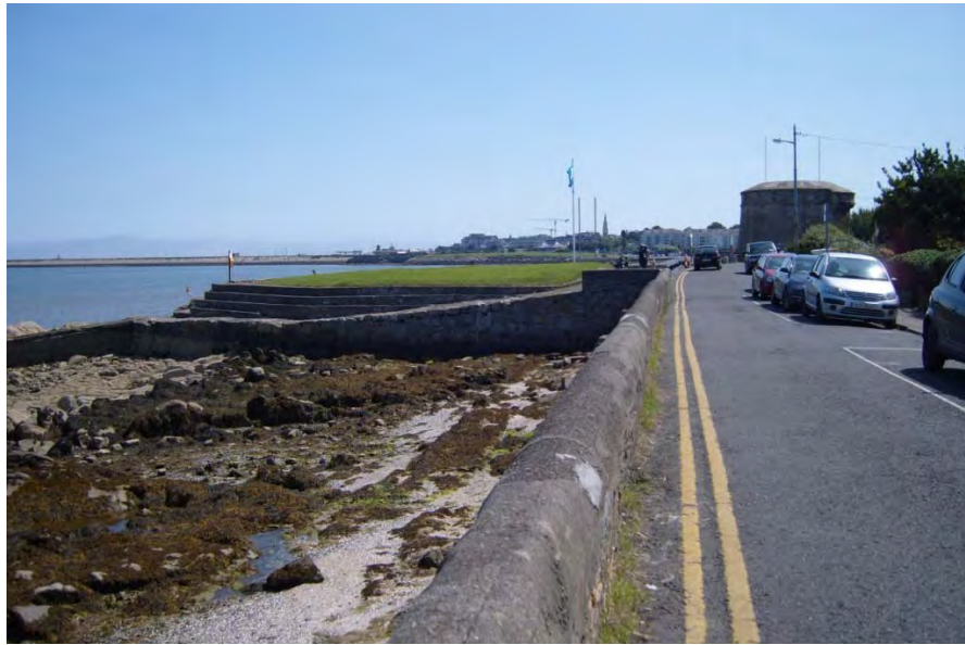
Figure 3.22 – View of Rocky Foreshore and Lawn Area to the North of the Main Bathing Area at Seapoint
