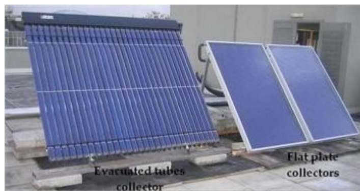
Figure 5.10. The solar thermal systems built and installed at a site in Dublin [63].
