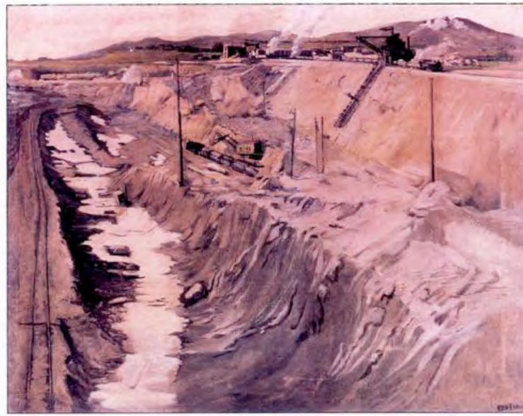
Figure 1.4; 'Building-site with Luffelbagger and Wagon Train' (source: ESB Art Portfolio Catalogue) Sean Keating
