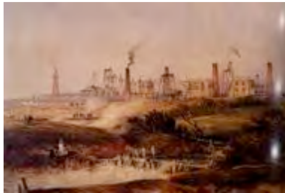
Figure 2.33; 'View to the Northeast, Murton, Newcastle Upon Tyne, 1841', Thomas Miles Richardson
