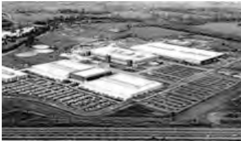
Figure 3.1; Hewlett-Packard (Manufacturing Limited) Liffey Park Technology Campus, Barnhall, Leixlip, County Kildare, 2002 (source: HP)
