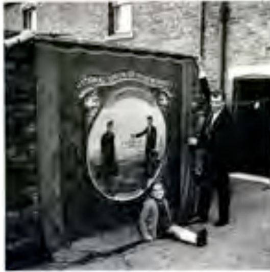
Figure 2.29; from Steelworks , photograph by Tommy Harris
