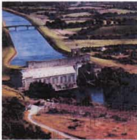
Figure 1.1; Ardnacrusha, County Clare (aerial photograph, ESB Archive)
