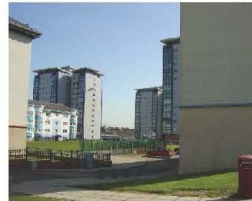
Multi-storey and low rise properties after improvement work
