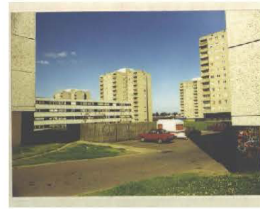
Multi-storey and low rise properties before improvement work
